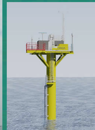
LIDAR System on offshore platform
