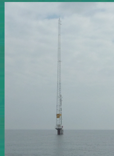
Wind Monitoring Mast
